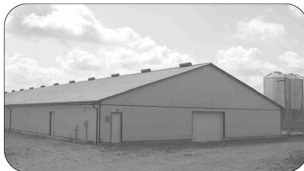
**Figure 4.** A naturally ventilated barn with chimneys through the attic space.
